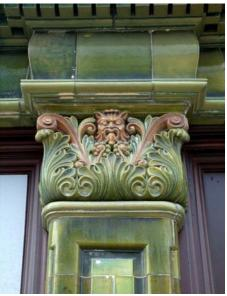
impervious and adaptable nature of glazed architectural terracotta. It could accommodate subtle nuances of modeling, texture and color. It never needed paint, and periodic washings restored its appearance from soot and other dirt.
